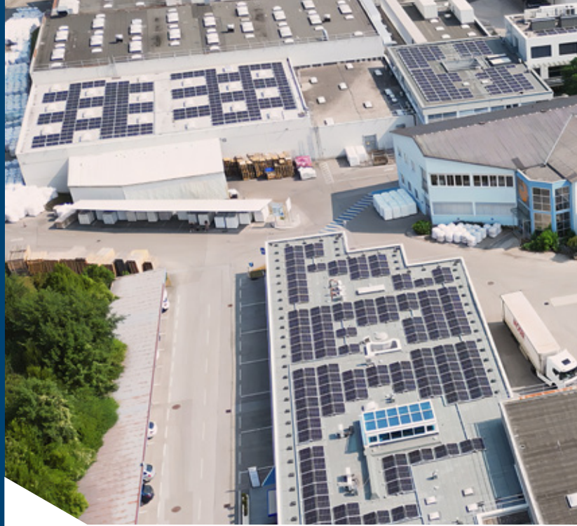
Photovoltaic systems at the Kremsmünster site
